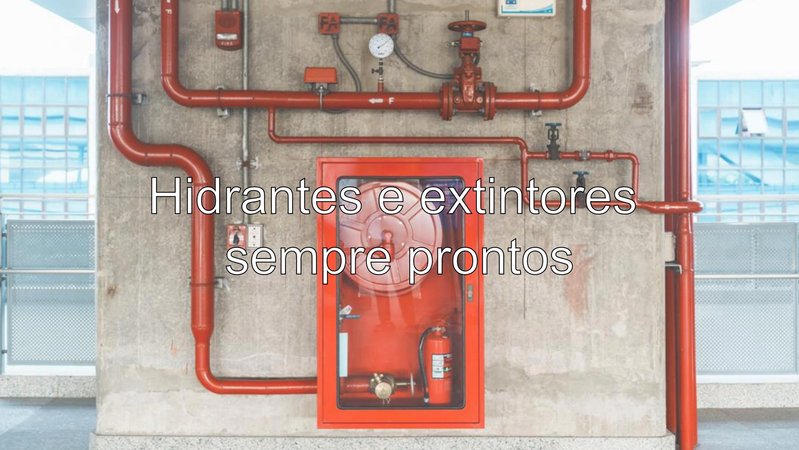
A photograph of a fire hydrant cabinet mounted on a concrete wall. The cabinet is red and contains a fire extinguisher and a fire alarm pull station. Above the cabinet, there is a network of red pipes, a pressure gauge, and a fire alarm control panel. The scene is set in a modern building with large windows and a balcony in the background.
